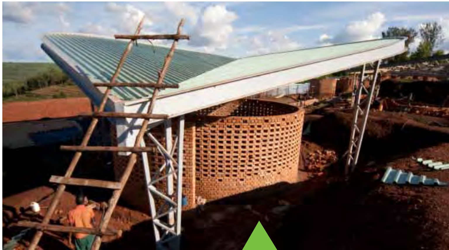
Above: The first of the center's seven classrooms under construction. The building's steel canopy serves as a rain collector. The perforated bricks walls allow for passive cooling and shading while providing a sense of privacy. Below: A series of solar studies for the roofs.
