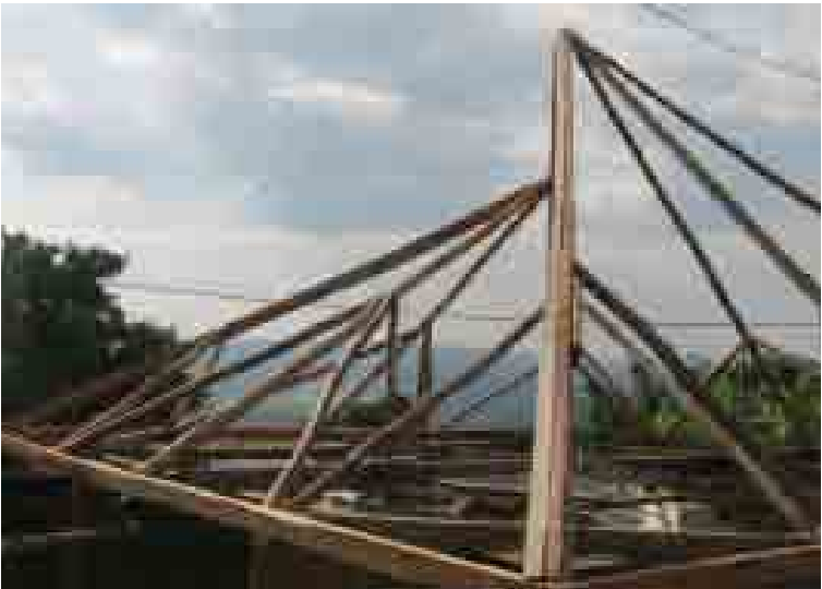
Our prototype: Roof framing made from local unmilled timber
