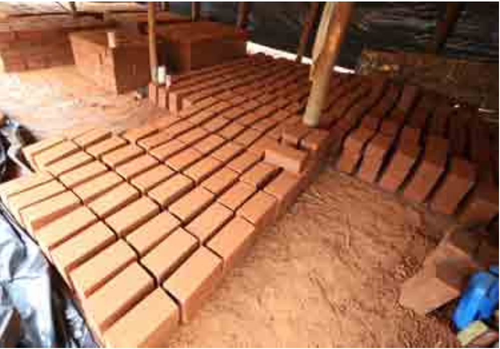
Compressed Earth Blocks produced on a large scale - Rwinkwavu Housing Project
