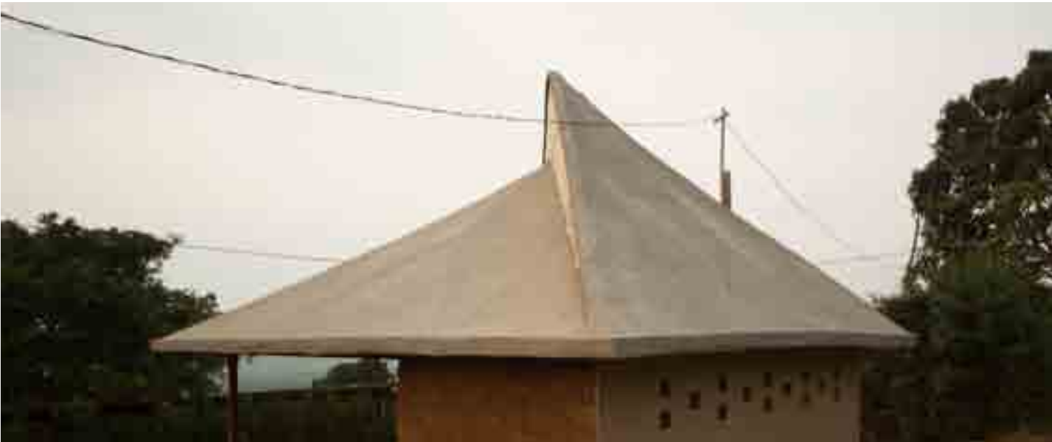
Our prototype: roof covered with a slurry of cement, latex, sand mixture
