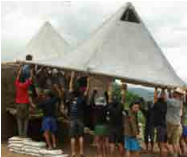
Precedent we learned from: easy to assemble on the ground and lift into place offering assembly line possibility
