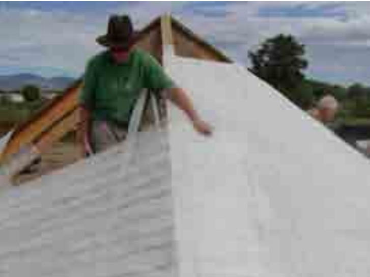
Precedent: roof form made from stretch mesh and chicken wire
