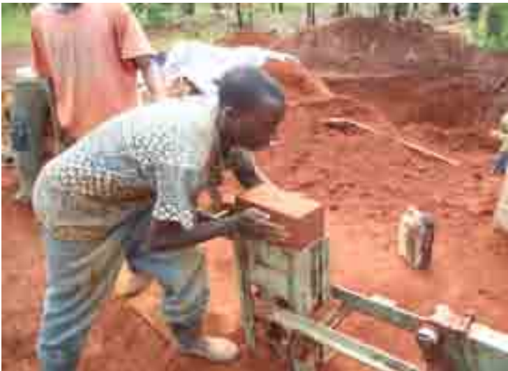
(4) Removing the block from the press
