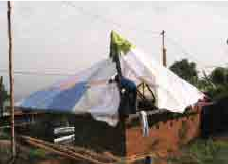
Our prototype: roof form made from old bedsheets and chicken wire
