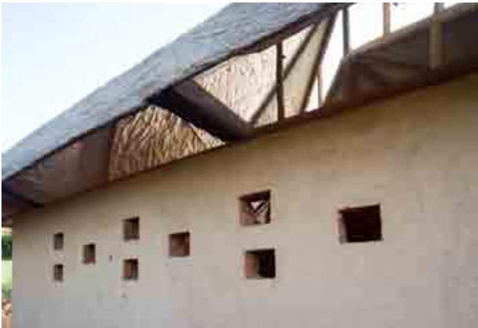
Ventilation at overhang of roof and in wall by subtracting blocks and adding insect mesh
