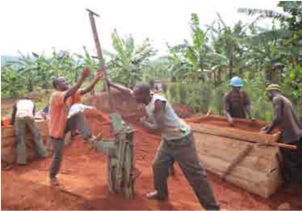
Local unskilled labour to produce Compressed Earth Bloacks - Rwinkwavu Housing Project
