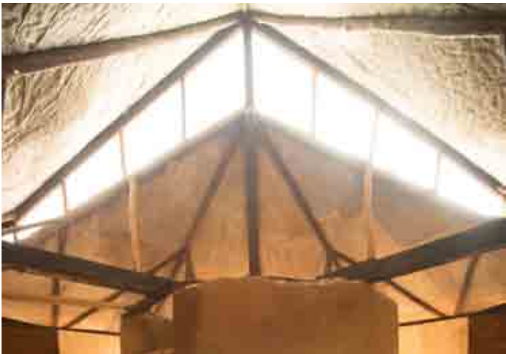
Natural Light and ventilation into the interior of the house - Rwinkwavu Prototype House
